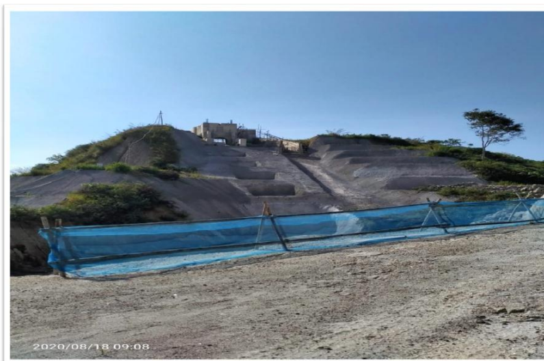
Figure 5: Mini-hydropower – Project Lau Biang (50.5% complete)
